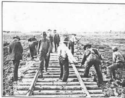
Track Laying on the First Railway to the Peace River Country.
